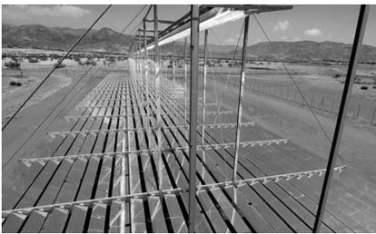
**Figure 7: Fresnel collector**
